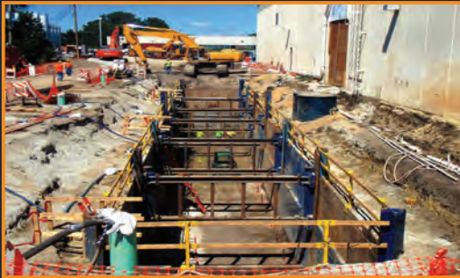
Slide Rail Shoring
